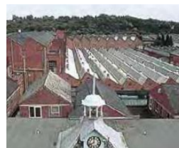
NSK Newark Plant
