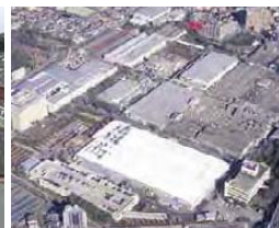
NSK Fujisawa Plant
